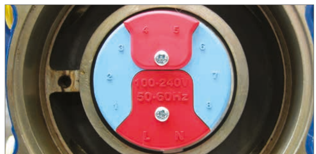
Fig 7.16 IS Terminal Block
